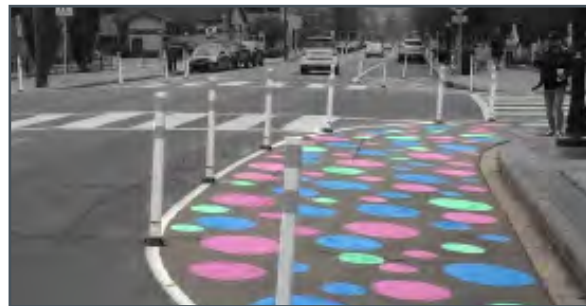
Temporary Curb Extension, Bridgeland, Calgary
